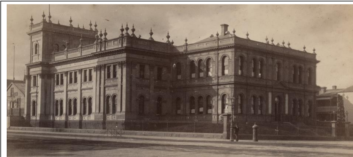
Trades Hall in 1889. Of the Lygon Street frontage only the southern part has been built. The central portico and northern part are missing. On the left-hand edge of this photo can be seen the original wooden hall built in 1859. (Photo: State Library of Victoria).
